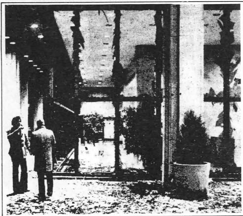
—Gulf and Western Building in New York City, bombed by FALN on February 18, 1977. One of the 4 sites attacked in N.Y.C. and Chicago to demand the immediate release of the 5 Nationalists a halt to the FBI's harassment of the Puerto Rican people, and warning against Ford's "Statehood" plan.
