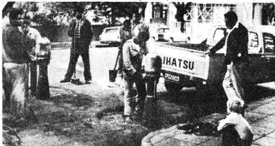
Construction workers in Pretoria.
