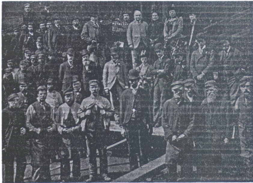
The workers of Laird Bros. photographed during the building of the "Royal Oak" at Birkenhead in 1890. Safety was accounted for. (From John Gorman's 'To Build Jerusalem' Scorpion Pubn.)
