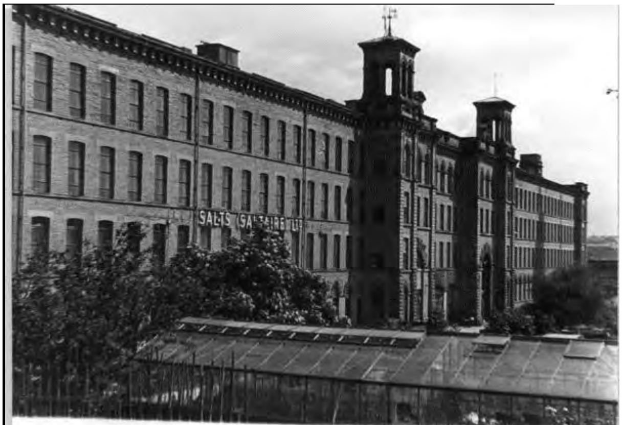
Salt's Mill, Bradford: the textile mill was built in 1851. Now it's a heritage centre... Photo: Workers
