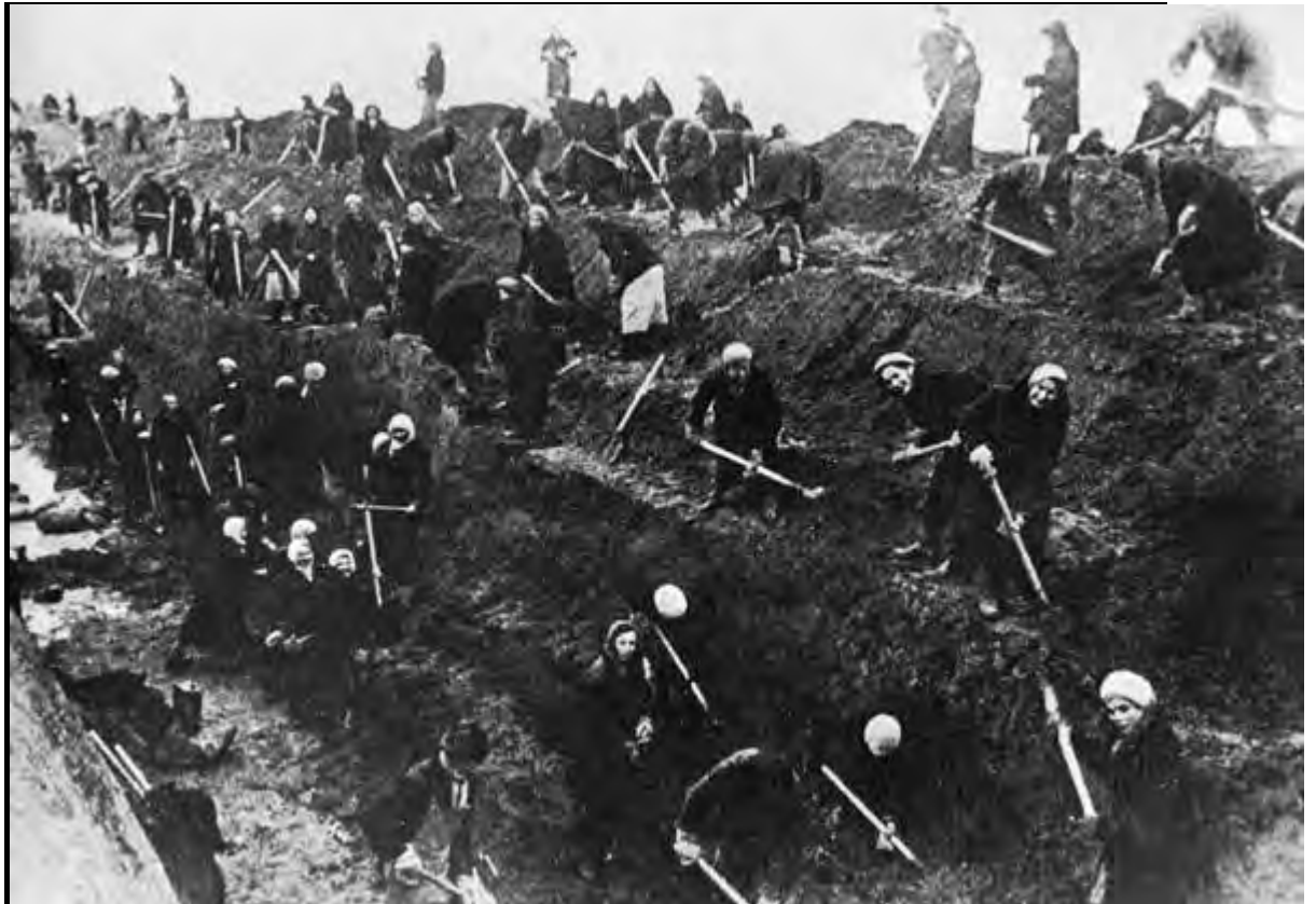
Armed with heavy shovels, Moscow women and elderly men build a tank trap to halt German Panzers advancing on the Russian capital. More than 100,000 citizens worked from mid-October until late November digging ditches and building other obstructions.
