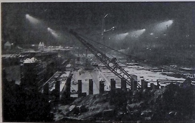
Building a new dock by night
