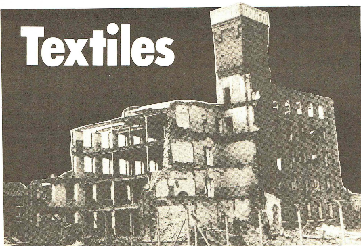
Townhead Mill, Rochdale; demolition, February, 1980
