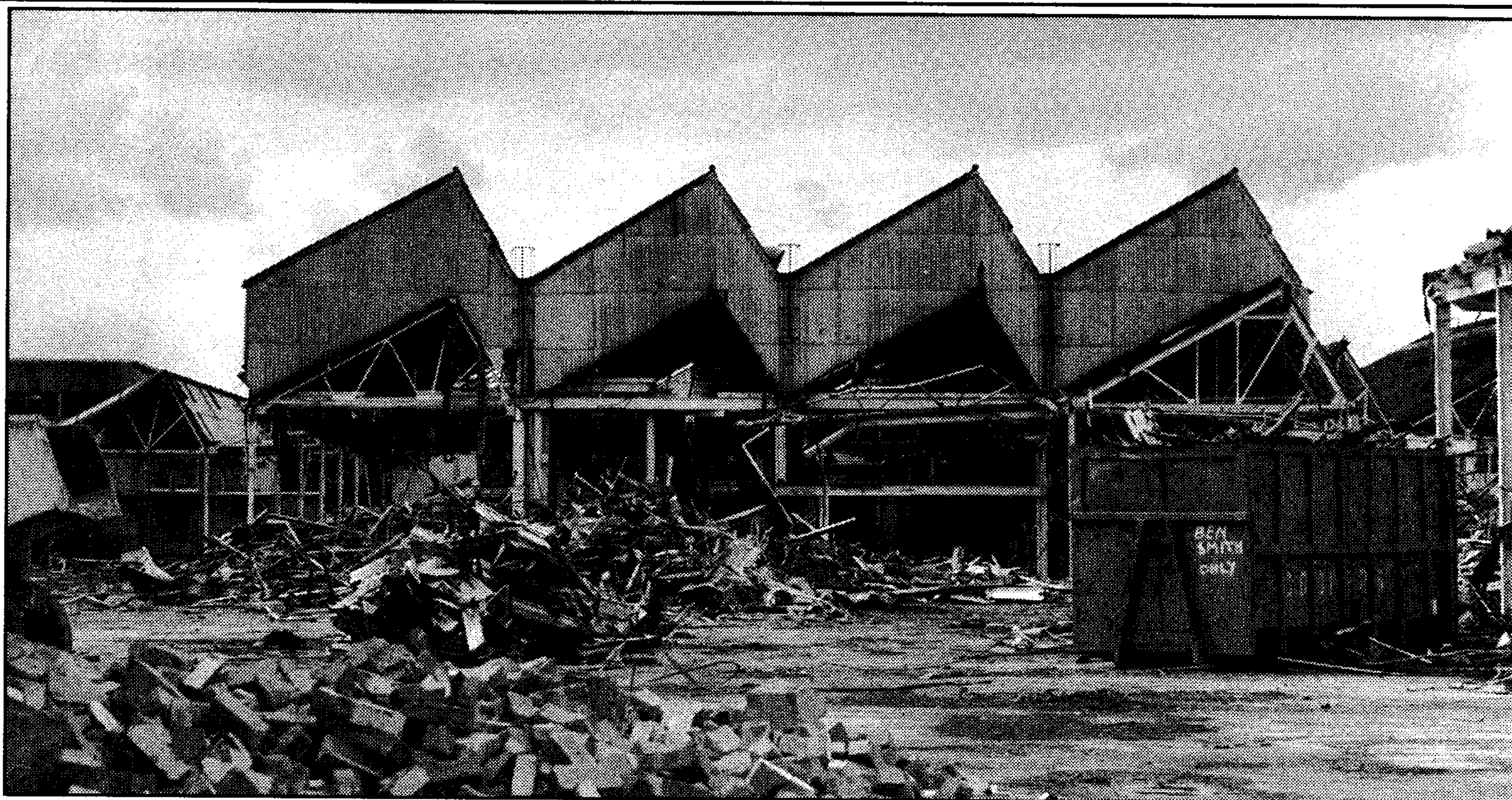
End of the line for more than half of Rover's Cowley works. What was the longest production line in Europe will give way to a Tesco's
