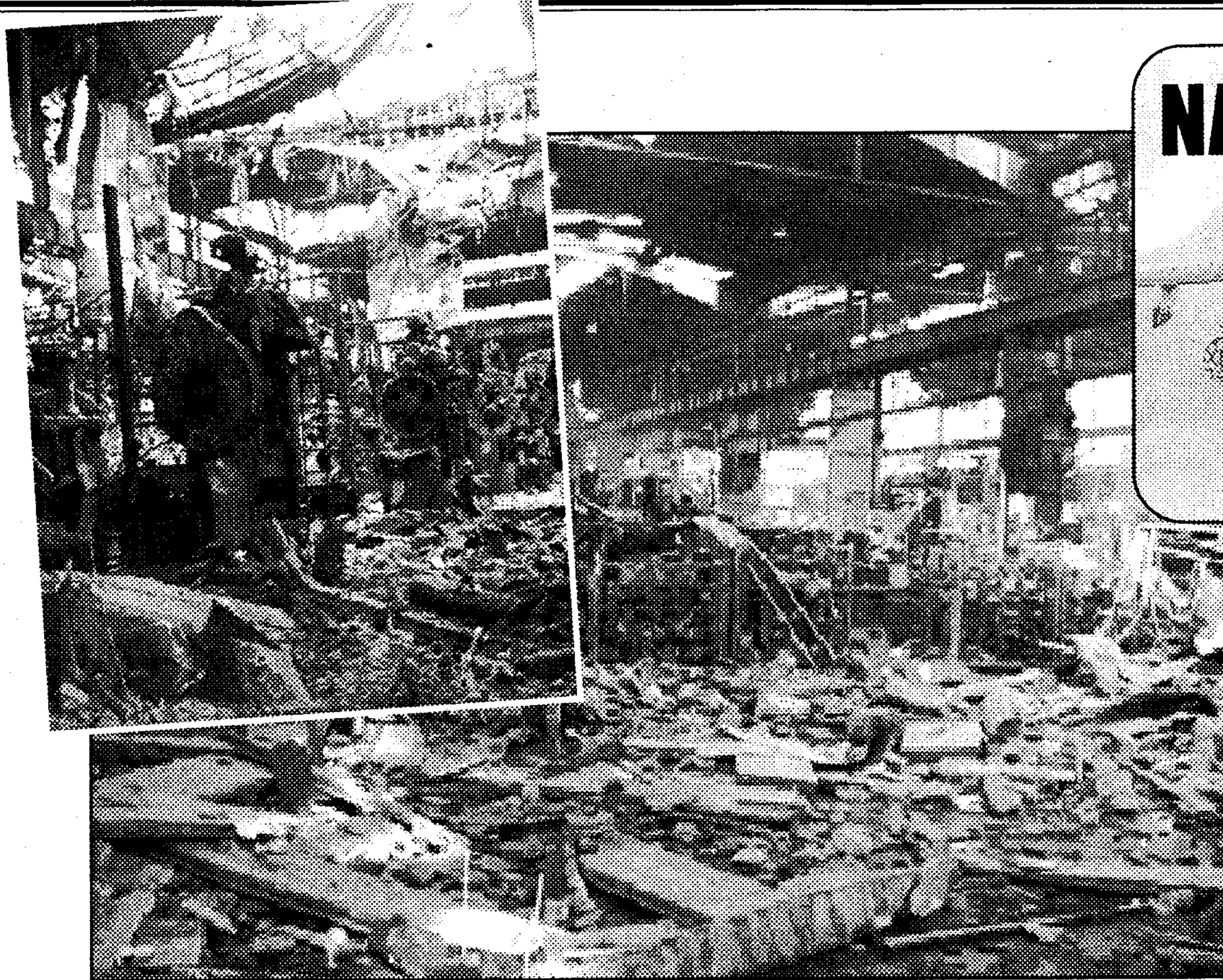
Demolished: the car plant where workers a year ago defied Milosevic
