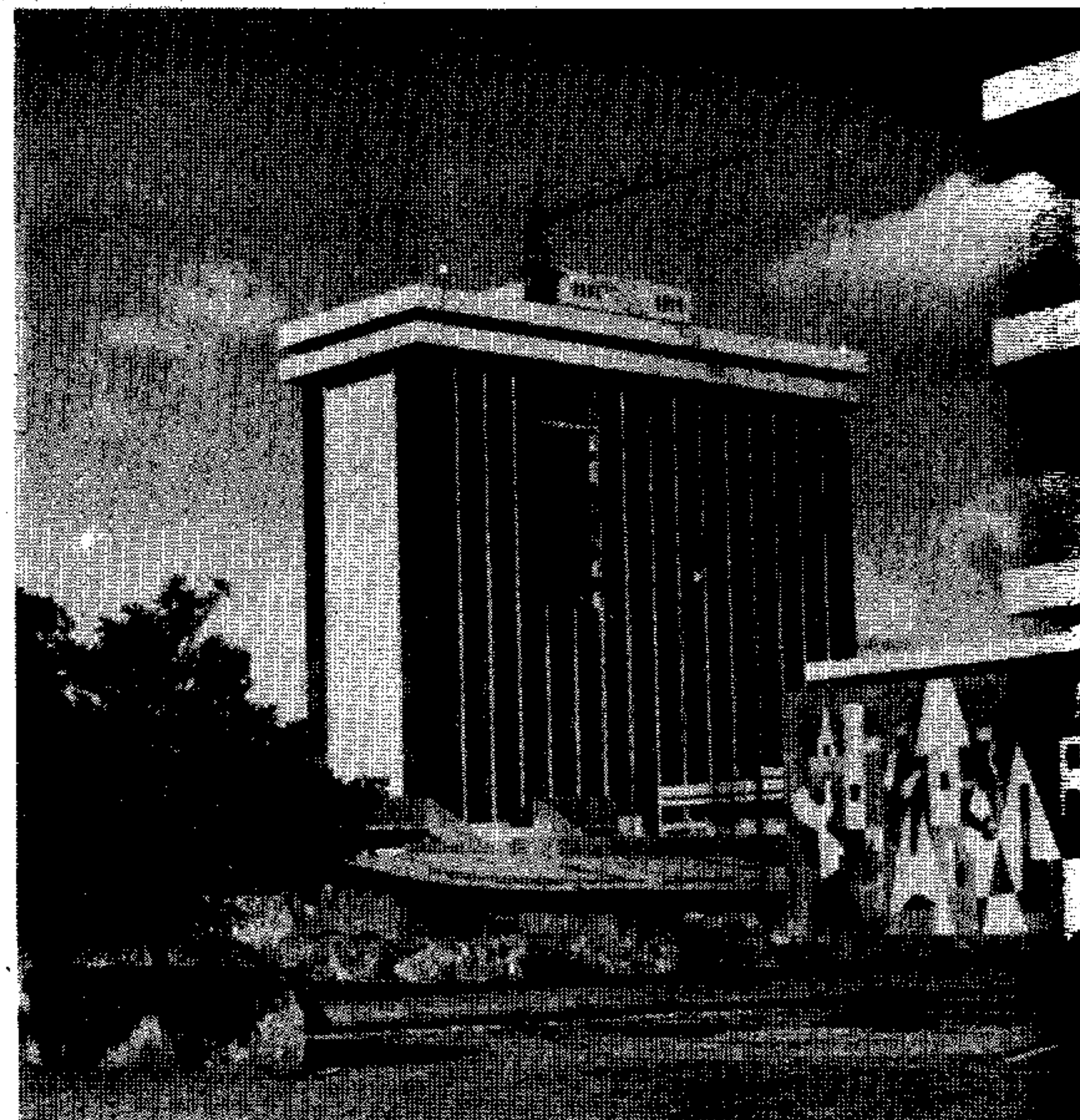
Unscathed after the Guatemala earthquake, the finance ministry building.
