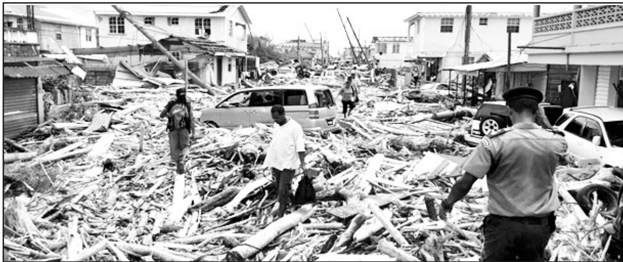
(Above) Storm-surge damage after Hurricane Maria hit the island of Dominica.
