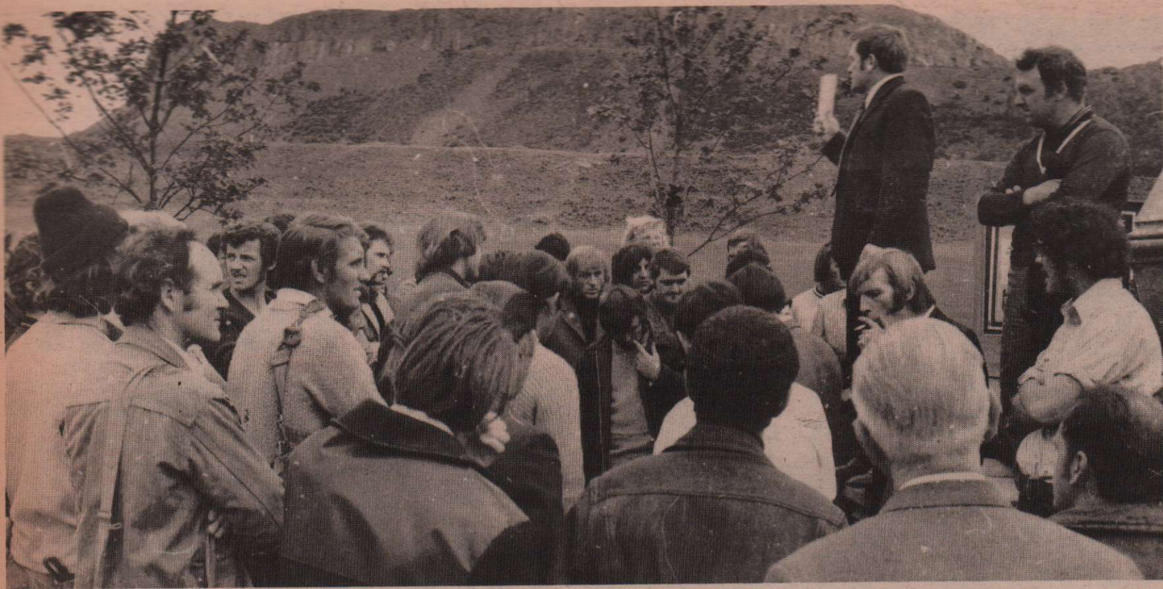
DURING the day, Bill Jones and Bob Williamson spoke at meetings on five building sites in the Edinburgh district. They spoke at Cameron's Moray House site, Myton's Dalkeith Road site, where Bill Jones is pictured above, McAlpine's St James Centre site, at Hart-Crudens in Livingstone and at the John Laing site for Heriot Watt University at Riccarton.
