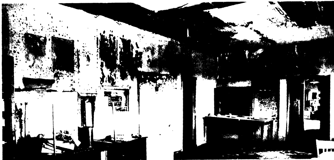
Photo indicating arson damage to SWP hall.
