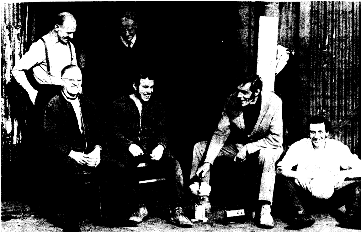
MEN INSIDE THE BREDBURY PLANT
