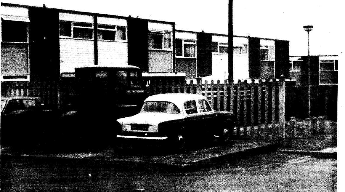
A newer part of the Bell Green housing complex on Coventry's eastern boundary now hemmed in by the Midlands link M6 motorway. But the design is the same—squares with houses facing in on each other—reminiscent of the 'greens' in Glasgow's Gorbals area.
