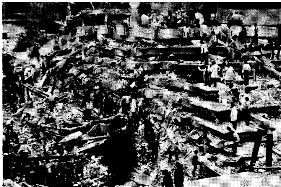
Earthquake damage in Mexico City, September 1985. More than a year later, 90,000 still lack permanent homes.
