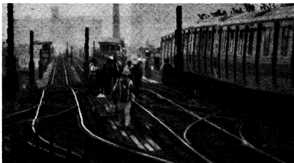
Gravesend, Brooklyn—Track where two transit workers were crushed by train.
