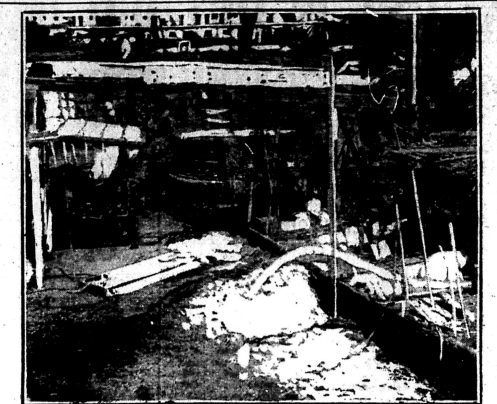
SCENE INSIDE THE IMMENSE COPPER DAM, WHERE THE OVERHAULING OF THE WRECKED BATTLESHIP MAINE IS GOING RAPIDLY FORWARD. A NUMBER OF SKELETONS HAVE BEEN FOUND. THE WATER HAS BEEN ENTIRELY DRAWN OFF AND THE PHOTOGRAPH SHOWS THE FLOOR OF HAVANA HARBOR.
