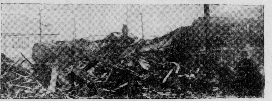
The ruins of a line of stores and houses in Detroit which were wrecked by an explosion. The explosion injured several workers and endangered the lives of all those in the city block.
