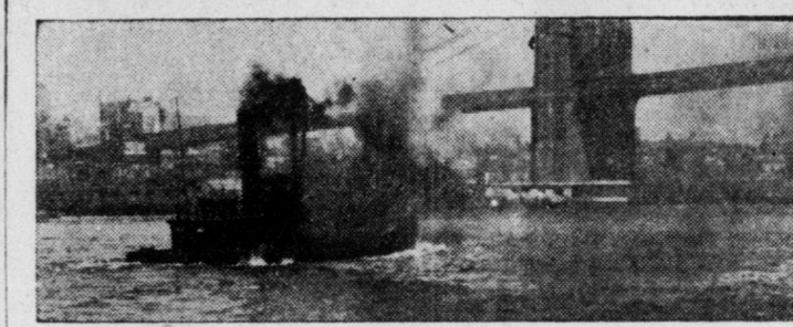
The lives of workers, working under great pressure on the new subway tube under the East River, were endangered when drills struck fissure in rock 80 feet under water. The leak was hurriedly plugged with cement by the workers, thus saving their lives. Photo shows bubbling water on surface of river caused by leak.
