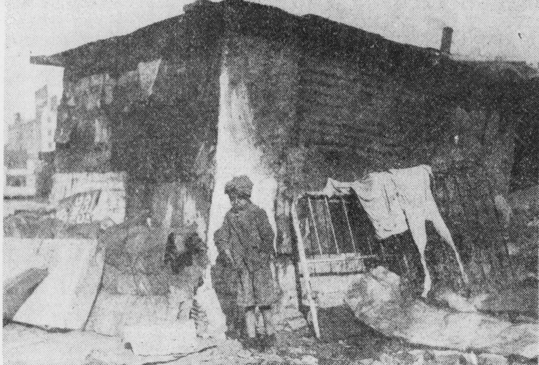
PART OF PARK AVENUE, seldom mentioned. Park Avenue, New York, is known as the street of millionaires, but a short walk from the homes of the wealthy parasites can be found this Negro worker's home and many others like it. A leaky makeshift shack of one room for the whole family. Outside stands one of the thin, ragged children, chief sufferers in the vile discrimination practiced against Negroes in jobs or relief.
