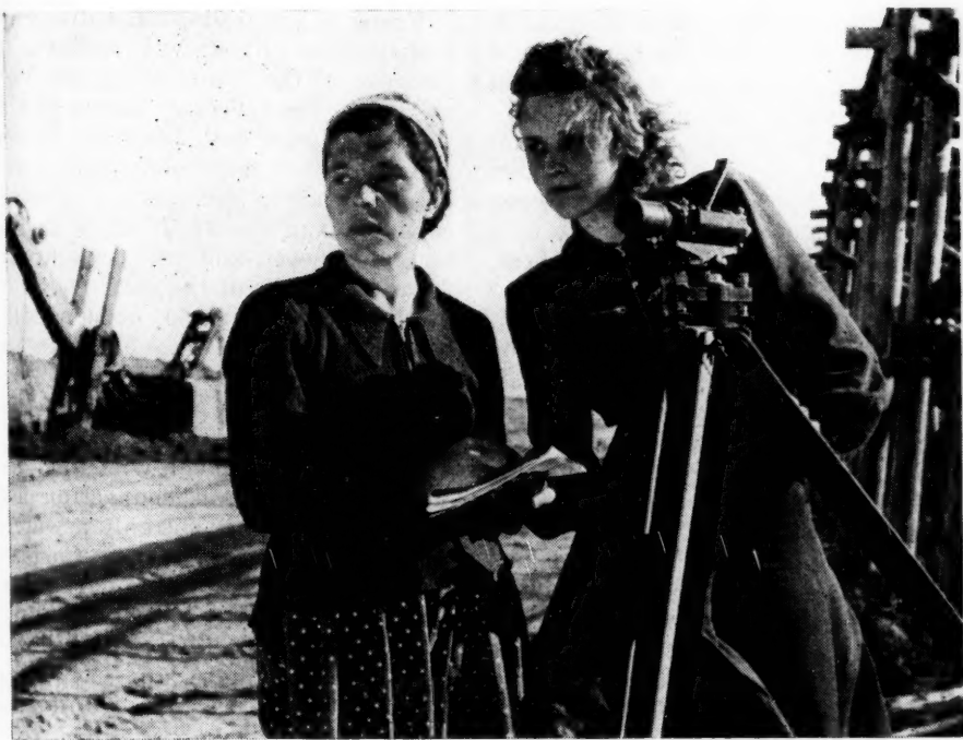
Geodesists survey the construction site of the Tsymlyanskaya hydroelectric station, part of the Volga-Don project connecting five seas
