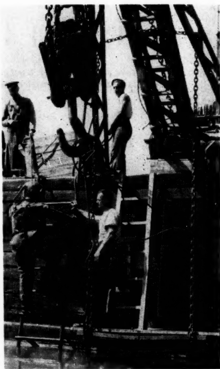
Divers descend into the river to work on the foundations of one unit of the Kuibyshev hydroelectric project
