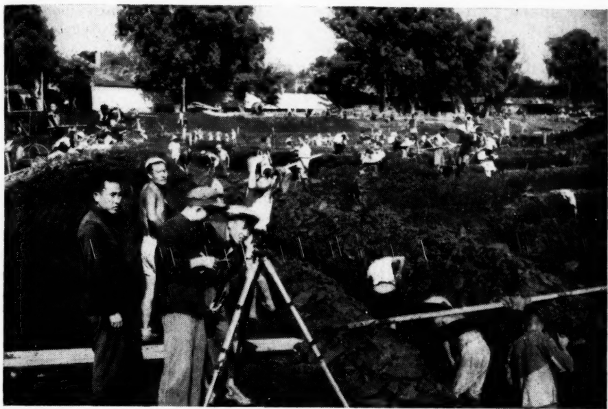
Building one of four swimming pools for a park in Peking which will also have other recreational facilities. The site is a former swamp, now drained and cleared
