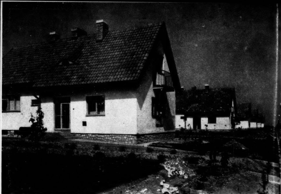
Some of the homes of the new Lidice (picture taken a year ago; landscaping is now completed). These homes, the water system and other public services, even the furnishings were supplied by State funds and contributions of Czech miners.
