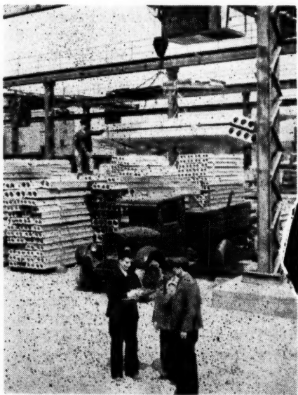
A crane loads pre-cast floors on a truck. Pre-fabrication has enabled Leningrad to speed its housing plan
