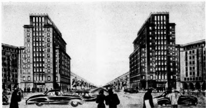
—Photos for this article from GDR in Construction Artist's drawing of Stalin Allee. Begun this year, some apartments are already occupied; the rest is to be completed before the end of the year
