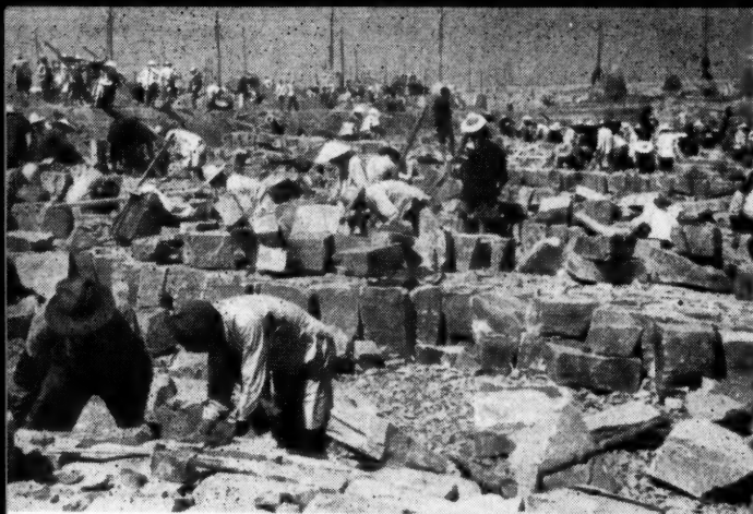
Stone masons working on the great project to prevent floods on the Huai. After centuries of destruction the river will be confined to its course
