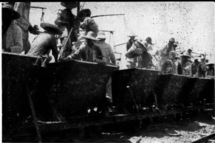
Workers on the Huai River flood control project load railway dump trucks used to convey building materials to the various construction sites
