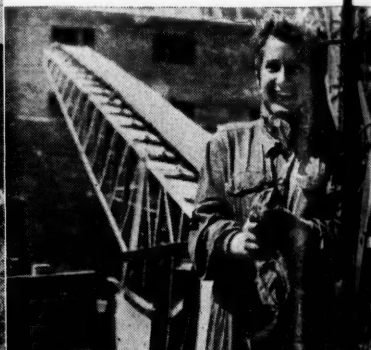
Margit Onodi operates a construction site of the Great Stalin Bridge.
