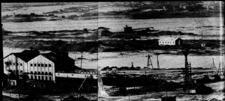
Construction site of the Angara Hydroelectric Station near Irkutsk, in Siberia. This is only one of several stations to be built on that river.
