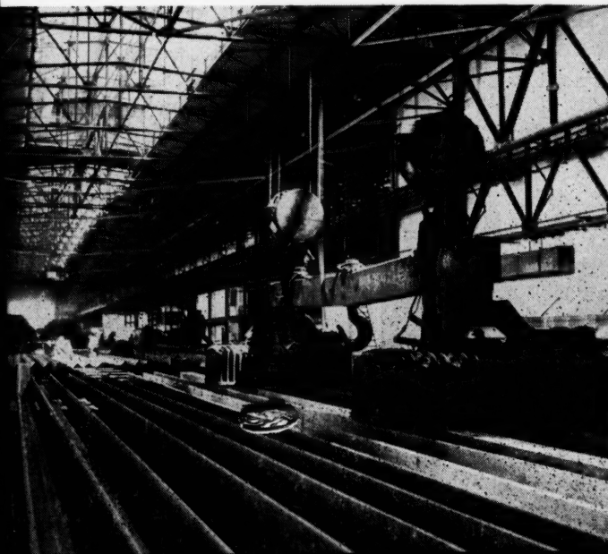
Steel for bridges made in the rolling mill department of the Anshan Iron and Steel Works in Northeast China
