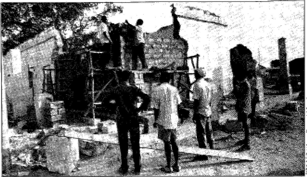
Angola resident rebuilds his destroyed house.
