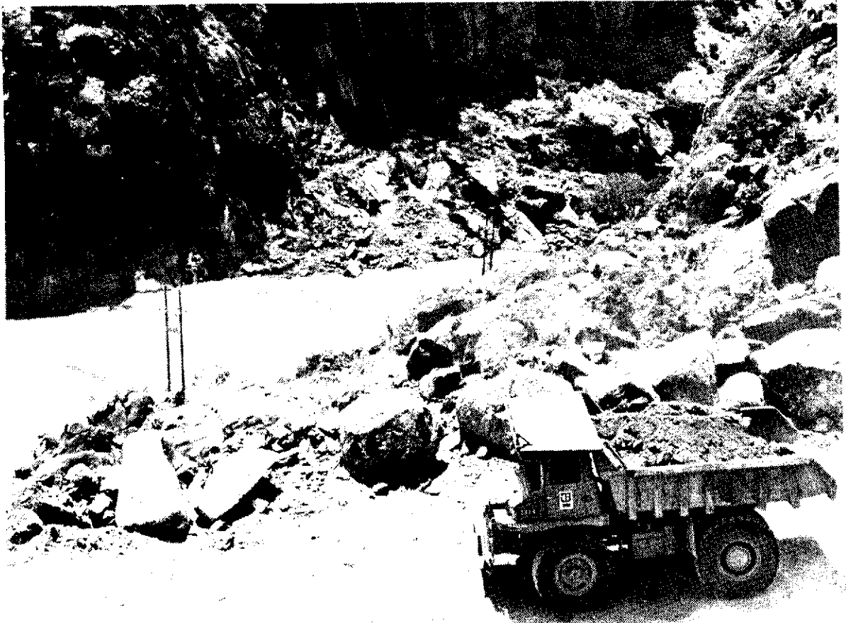
Construction work at the Cabora Bassa dam site.
