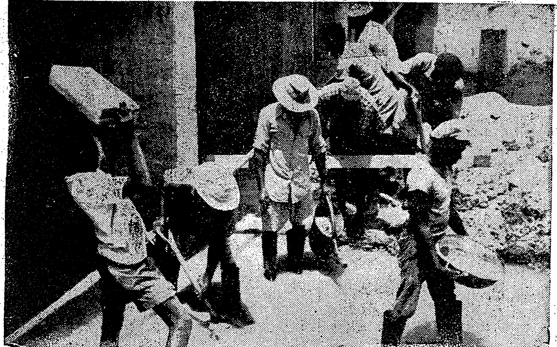
Workers of Housing Corporation seen busily building a house
