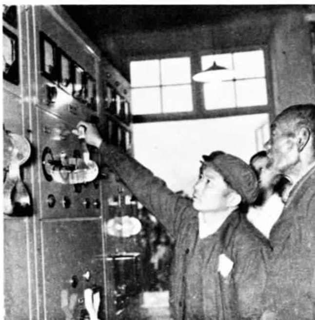
At the power station in Shigatse
