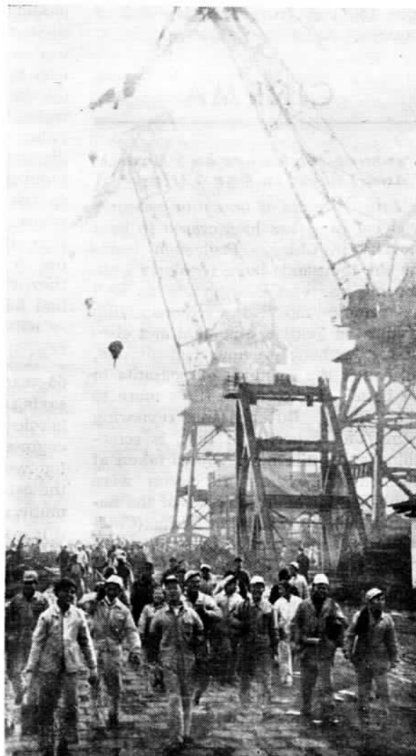
Off to Work in the Morning
