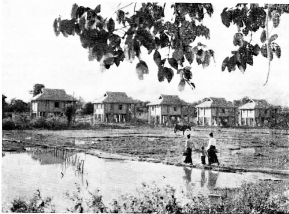
Newly built houses for the Tai people in Yunnan Province
