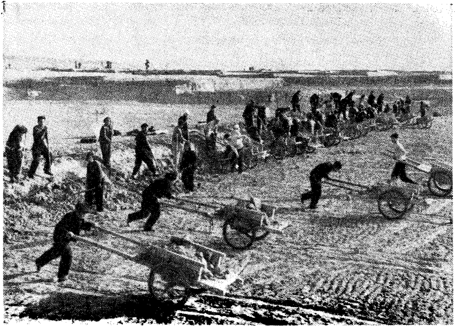
Rebuilding a terrace embankment
