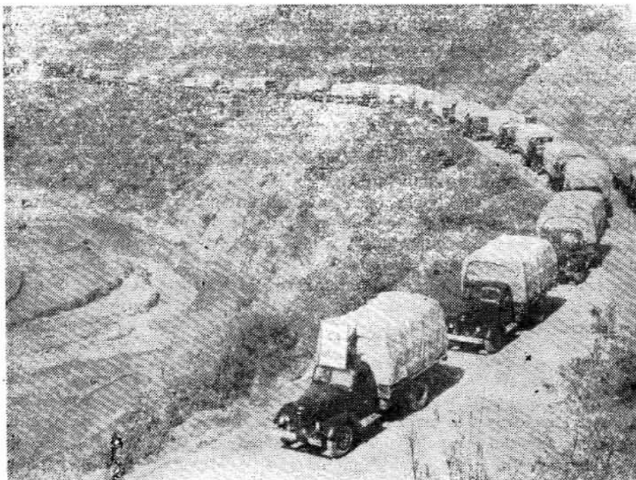
A new highway is open to traffic.
