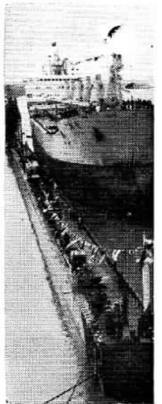
The 25,000-ton floating dock Huangshan built in Shanghai.
