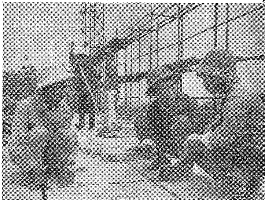
Students learning construction management at a work-site.
