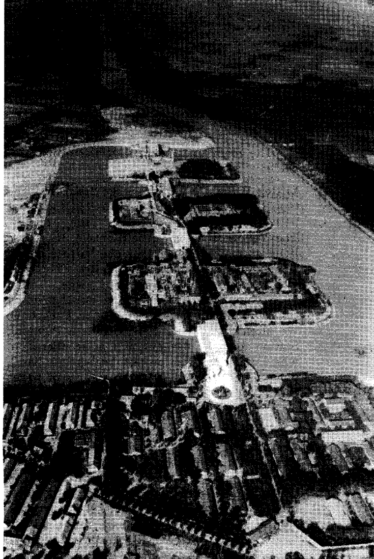
Chiangtu Pumping Station.
