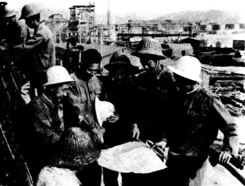
Power plant work-site in Shantung Province.
