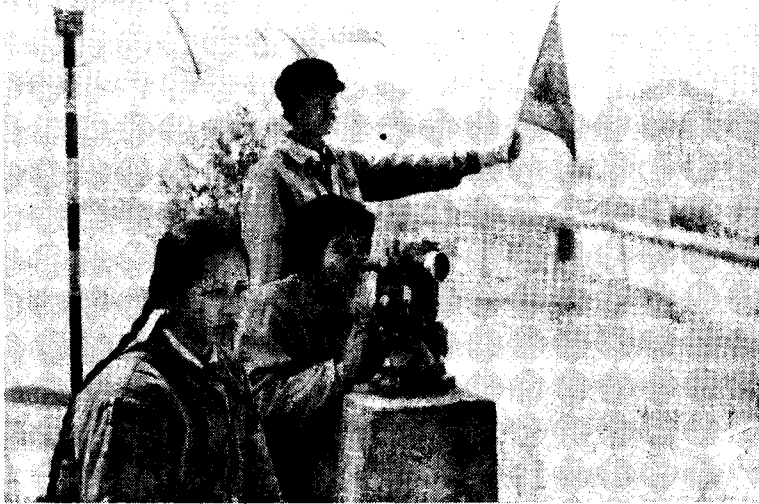
Surveying, Huanghe River work-site.
