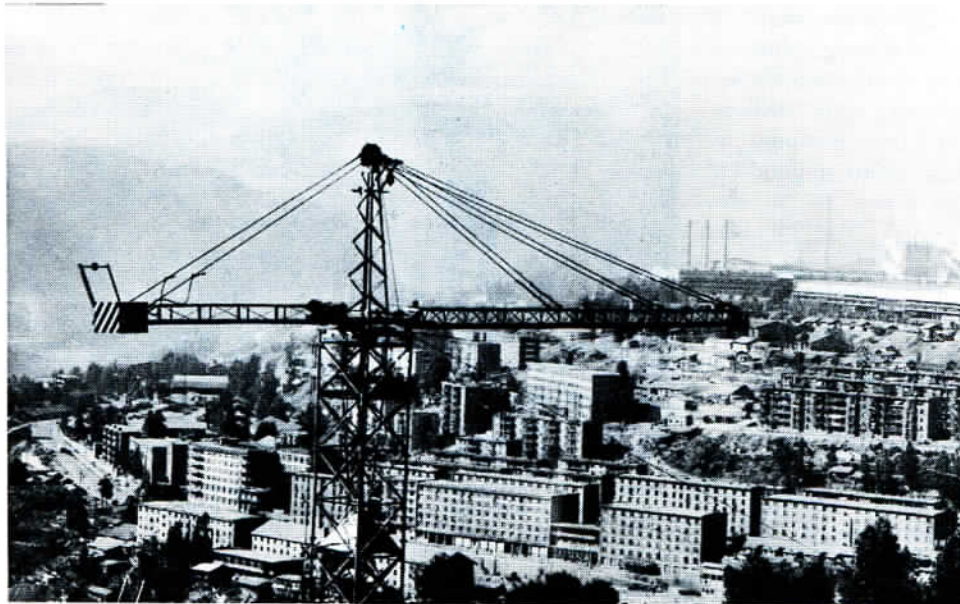
Housing construction in Dukou, a new industrial city in Sichuan Province.
