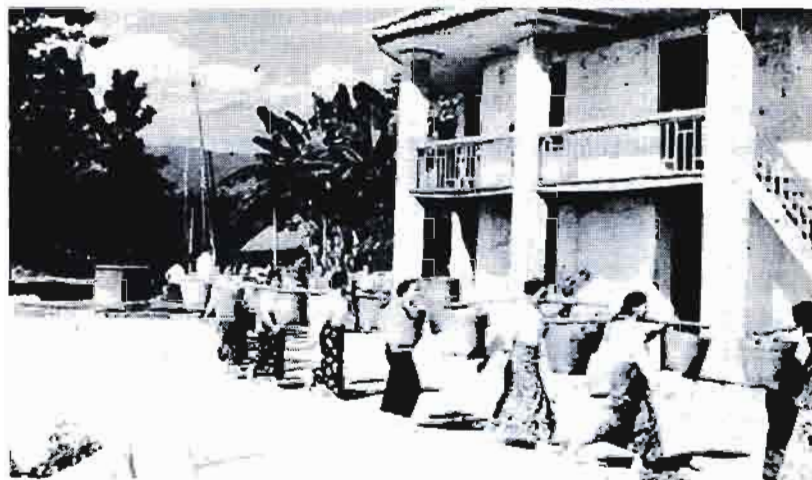
The Dai people who used to live in simple bamboo houses often suffered from accidental fires and insect pests. Now two-storeyed brick buildings with verandas have been built in some places. This is a new building of a Dai nationality village in Yunnan Province.
