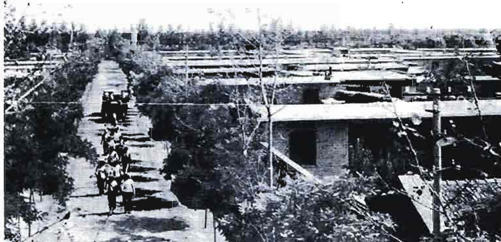
Flat-roof brick houses, typical peasant houses on the north China plain, are built with less work and materials. The roof can be used as a sunning ground. This is a new village built in Hebei Province after the earthquake in the Xingtai area in 1968.
