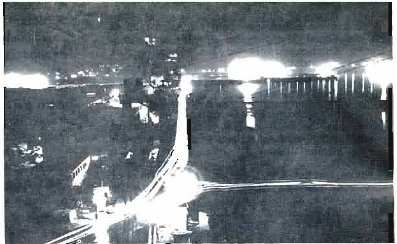
The Gezhouba work-site at night.
