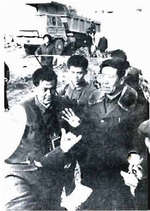
Liu Shutian (centre), who directed the damming of the river, at the work-site.
