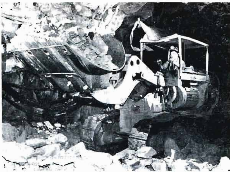
Tunnelling in a coal mine in Anhui Province.
