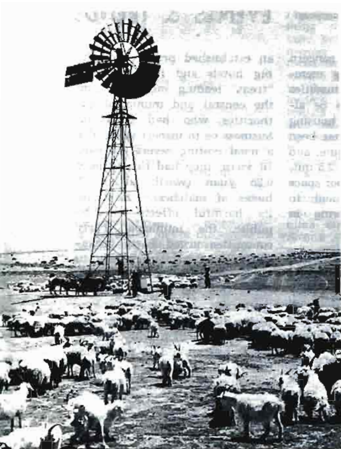
A well operated by wind power on the Inner Mongolian grassland.
