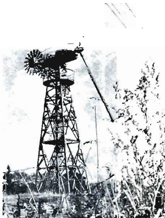
The wind power generating unit designed by the Heilongjiang Machinery Research Institute.
