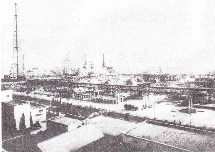
The Shanghai Petrochemical General Works in Jinshan County.
