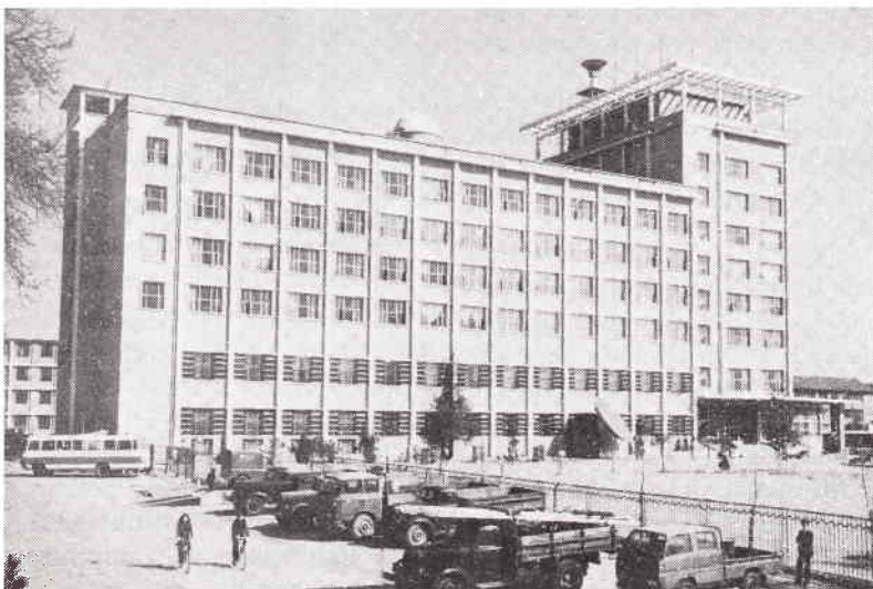
The National Meteorological Centre in Beijing's western suburbs processes data from all corners of the world every day. It is also one of the key meteorological centres in Asia.
