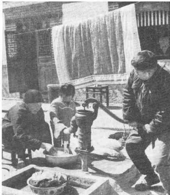
A hand-pumped well built by peasants in Yexian County, Shandong Province. Water and environmental sanitation in the county is highly valued.
